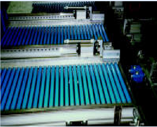
Roller conveyors combined with belt conveyors, stops and pusher stations.
